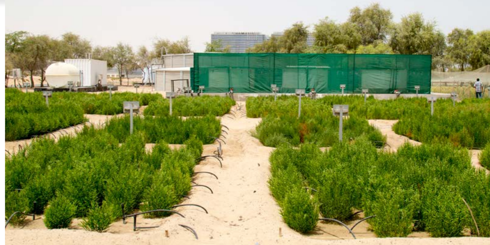
The Integrated Aqua-Agriculture System at ICBA is designed to maximize use of water for high-value and salt-tolerant crops, as well as fish species.
